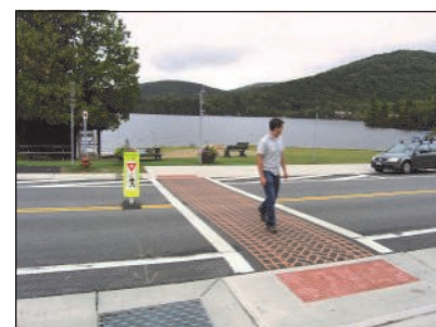
A new Complete Street in Blue Mountain Lake
